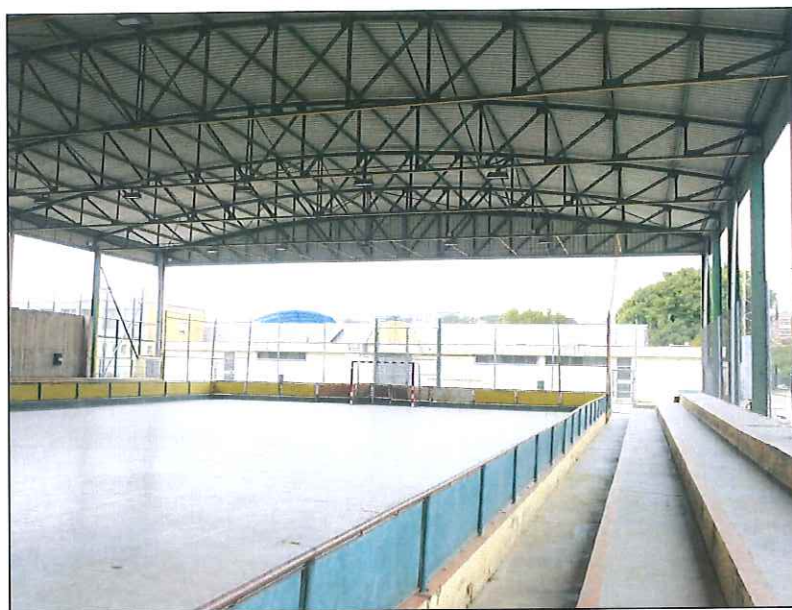
Vista 3 - Vista interior
